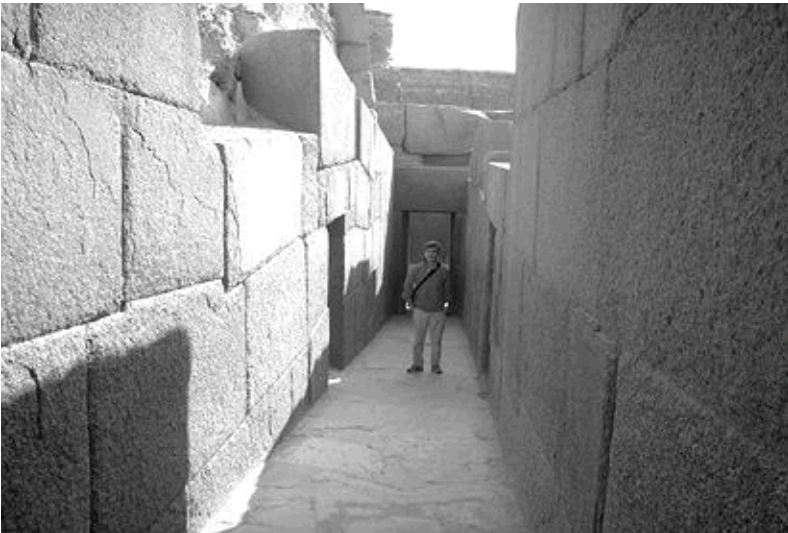
Figure 17b: Stage 17, Khafra Valley Temple (inside), casing made of small granite blocks with fine flat exterior surface and irregular belly shape in contact with the limestone core (1988).
