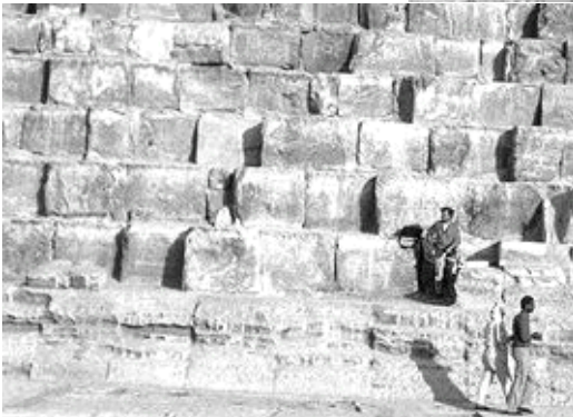
Figure 1c: (bottom) unweathered blocks protected by sand (1984).
