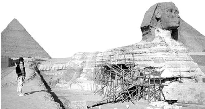
Figure 18a: The Sphinx seen from the Khafra Causeway, head made of hard grey Mokattam Formation, body resulting from quarrying the soft marly yellowish limestone (1988).
