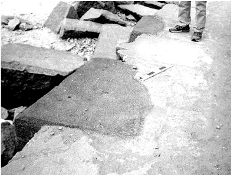
Figure 4: Irregular granite blocks on the west side of the Second Pyramid suggest builders of the Fourth Dynasty were unable to quarry regular granite blocks, if these were part of the original masonry.
