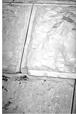
Figure 71 (right): Even with modern steel tools, dressed casing blocks did not provide close fit rather a gap up to 0.5 cm (0.2 inches) wide, and chipped corners.
