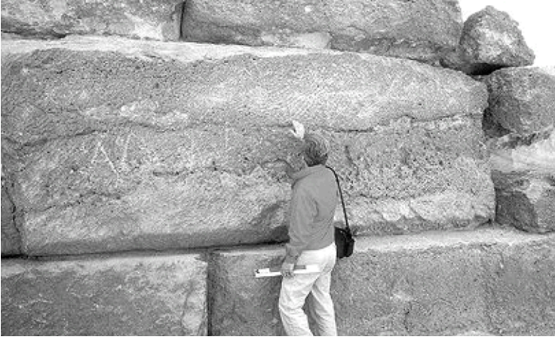
Figure 30a: Stage 11, Mortuary Temple, Menkure (Mykerinos) Pyramid, east, on the right hand when facing the valley. Blocks with tool-marks for plaster adherence and worked edge (1988).
