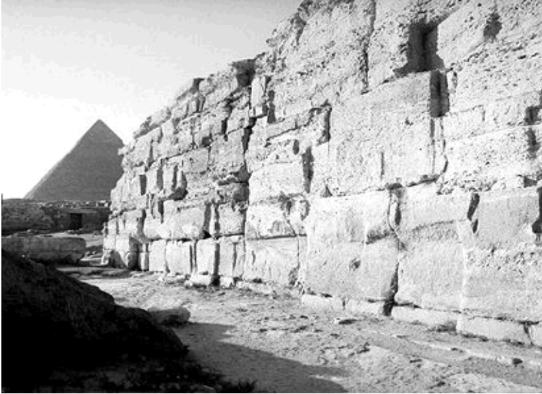
Figure 17c: Stage 17, Khafra Valley Temple (south side), limestone surface represents the negative face of the granite claddings (1984).
