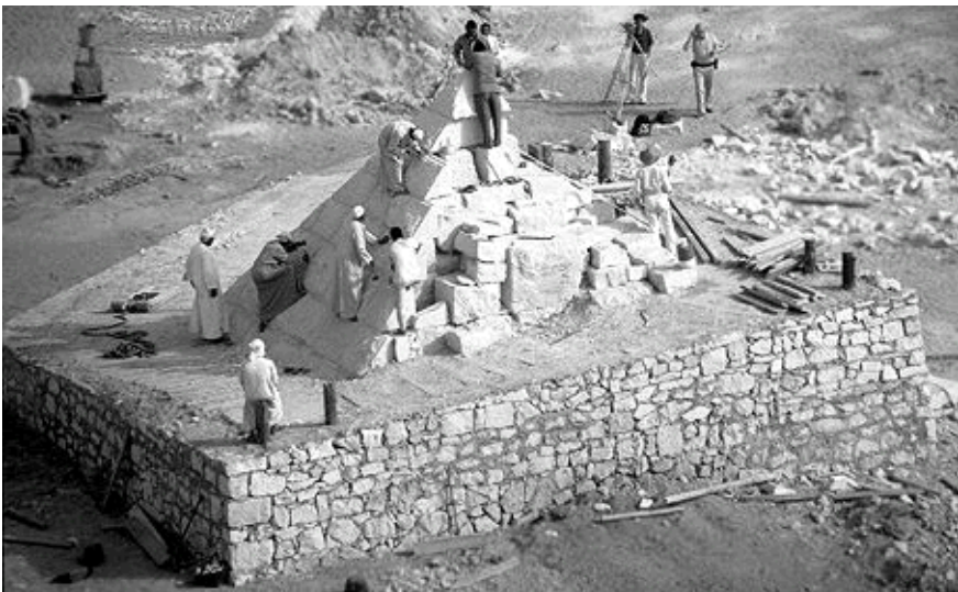
Figure 74: NOVA mini-pyramid and its gigantic wraparound ramp demonstrate the difficulty of the ramp scenario with its enormous amount of material (1991).
