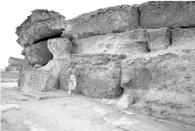
Figure 27: Enormous blocks in the mortuary temple of Khafra exhibit lightweight, weathered top portions characteristic of concrete (1984).
