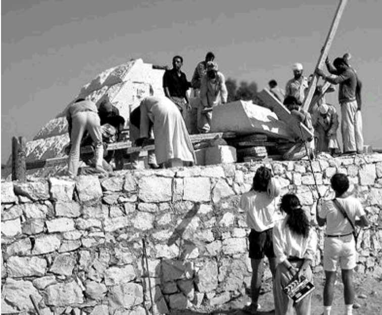
Figure 73: NOVA crew (foreground) filming the desperate efforts of lifting one stone block with wooden levers. It took 5 hours to lift the stone from ramp level to top level.
