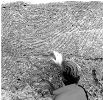
Figure 11b: visible toolmarks (1988).
