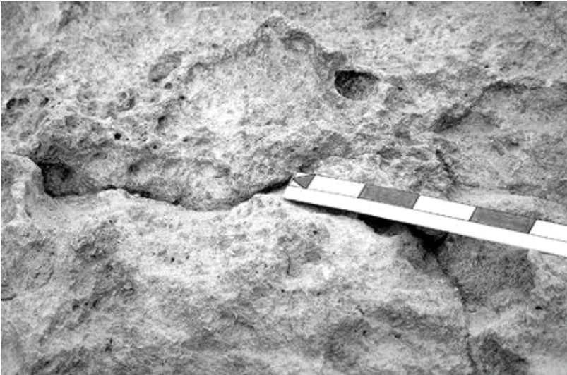
Figure 28: Blocks at Khafra's mortuary temple have wavy lift lines characteristic of construction interruptions during casting (1984).
