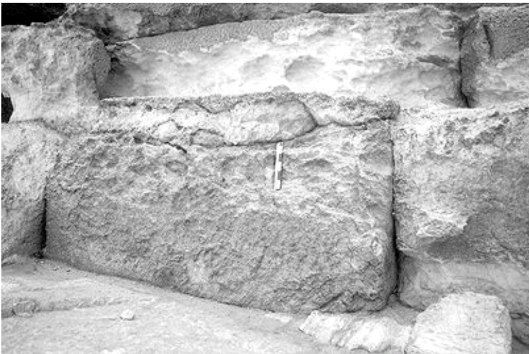
Figure 9: Stage 9, Mortuary Temple, Khafra Pyramid east. Block with strata, on right hand when looking east, to the valley. Notice the close vertical fit between the blocks and the thin mortar separating each block (1984).
