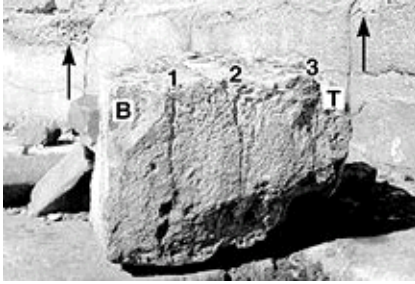
Figure 22: Block fallen from southwest corner of Khafra's pyramid has three lift lines (B-bottom; T-top); behind arrows show weak top layer (1984).
