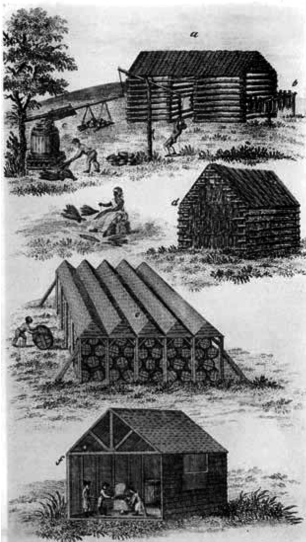
a, The common tobacco house. b, Tobacco hanging on a scaffold. c, The operation of prizing. d, Inside of a tobacco house, showing the tobacco hanging to cure. e, An outside view of a public warehouse. f, showing the process of inspection.
