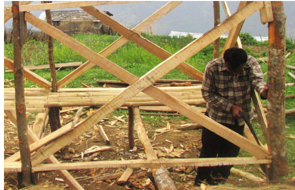
Fig. No. 2.4.3.1 Constructing earthquake resistant goat shed using cross beam
