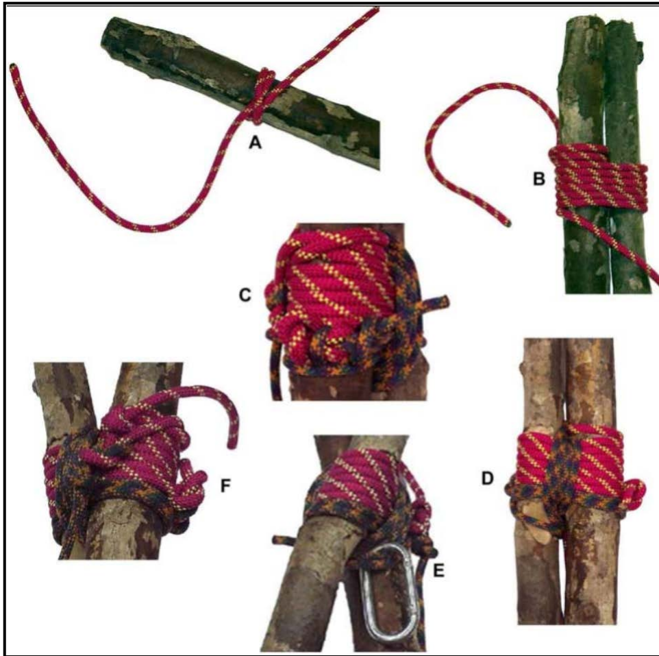
Figure 7-20. A-frame horizontal and vertical wraps.
