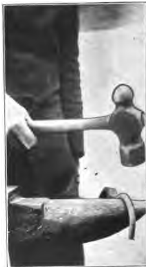
FIG. 13. BENDING OVER THE HORN OF THE ANVIL.
