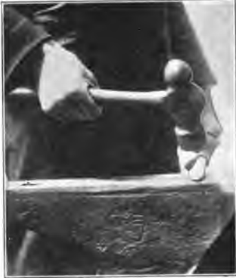
FIG. 42. FIRST STEP IN SHAPING A SCARF.
