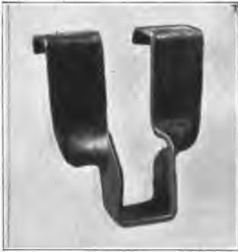
FIG. 36. JOIST STIRRUP.
