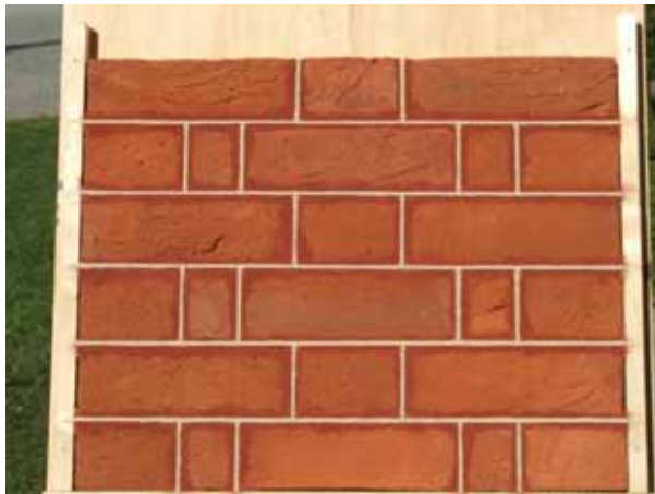
Figure 5.20: Trial Panel 03 Tuck pointing
