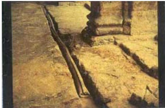
This lead pipe was made by hammering sheets of lead around a wooden pole.
